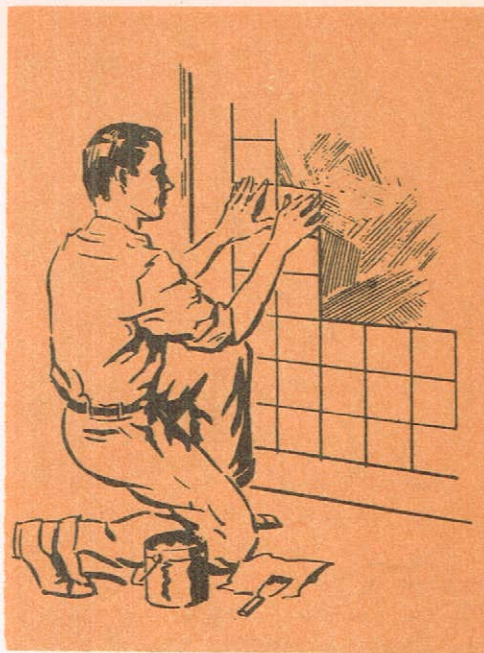
Fig. 33. Metal or plastic tile can be installed before or after the fixtures have been installed.
