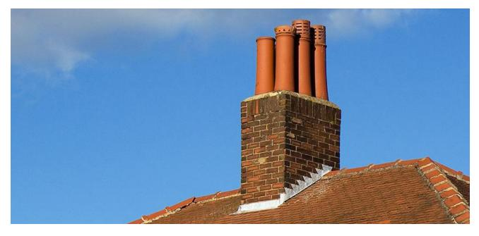
One of the most common <u>internal alterations</u> carried out is to remove an obsolete chimney breast at ground floor to create more floor space. Quite often the chimney is also removed at first floor level leaving just the roof void and external section of the chimney in place. Building Regulations apply to this work because it is a 'material alteration' to the structure ensuring the remaining part of the stack is properly supported.
