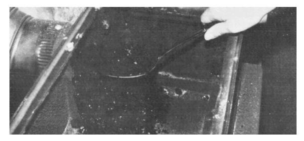
To clean prefabricated chimneys, many stove dealers sell round wire brushes which can be attached to small diameter metal pipes or ropes. The pipe or rope with the brush attached is then moved up and down in the chimney until all creosote deposits are removed. The deposits should fall to the bottom of the chimney and must be removed (Figure 6). Although not as effective, burlap bags filled with straw and weights such as rocks can be pulled up and down the chimney to remove creosote deposits.
