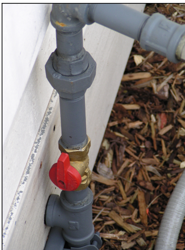
Figure 2-5 Manual Fuel Shutoff Valve (outdoor installation shown)
