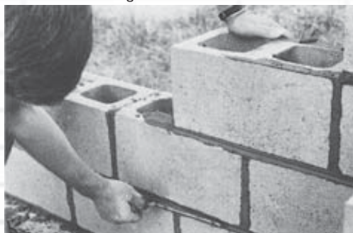
Tool horizontal joints
