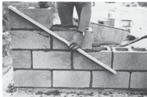
Check corner alignment
