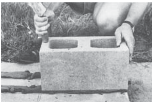
Tapping the block into position
