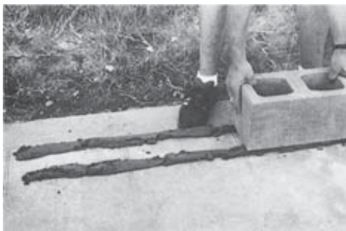
Positioning first corner block
