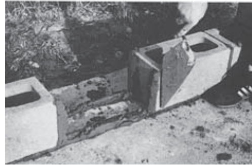
Mortar for closing block
