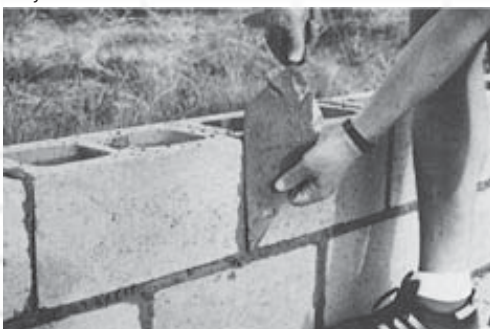
Re-fill mortar joints
