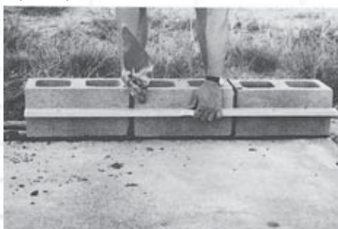
Check alignment with straightedge
