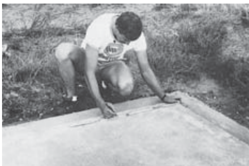
Setting out to block modules
