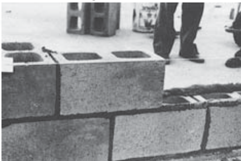
Lay blocks to mason's line
