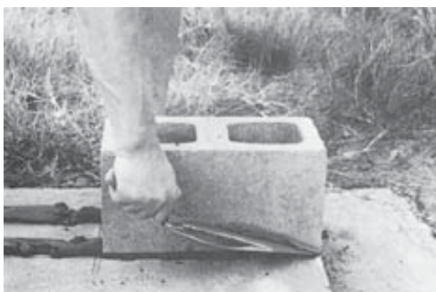
Remove excess mortar
