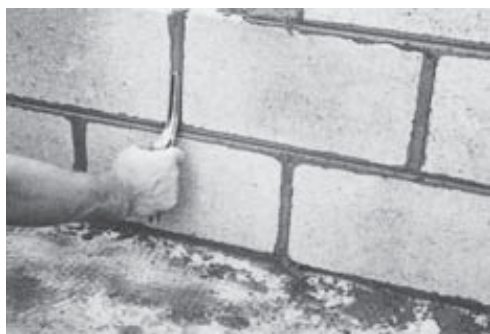
Tool vertical joints
