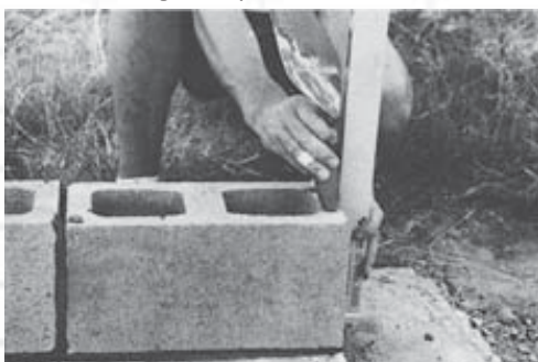
Check corner for plumb
