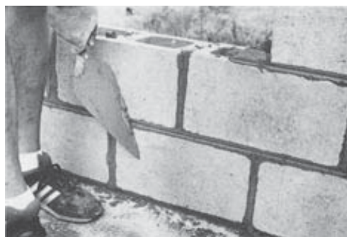
Remove excess mortar burrs
