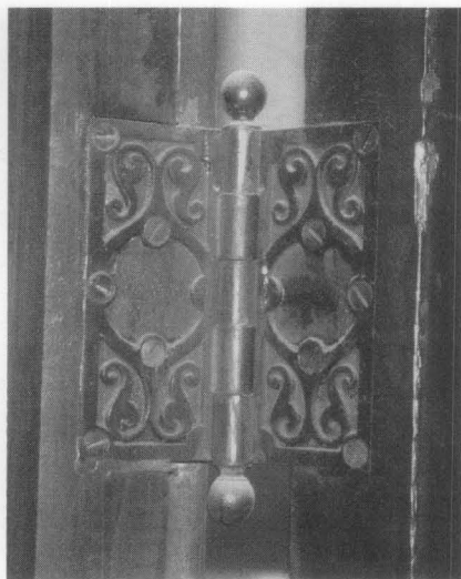
Figure 6. Original hardware including doorknobs, escutcheon plates and hinges were retained. Photos: McClier.
