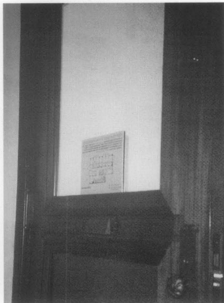
Figure 4. View of a Reliance Building office door from inside guest room. Upper and lower door panels have gypsum board secured to back with new molding. A mirror was affixed to the upper panel while the lower panel was painted to match original material. Photo: Chad Randl.
