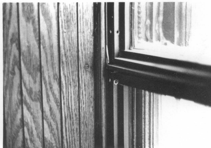
Figure 6. The windows were too large for only a single storm panel, necessitating the use of a structural subframe at the mid-section of the window. Both the upper and lower storm panels are operable and come together opposite the historic meeting rail. This element of the storm window is sufficiently thin that is not readily discernible from the outside. Photo: Charles E. Fisher
