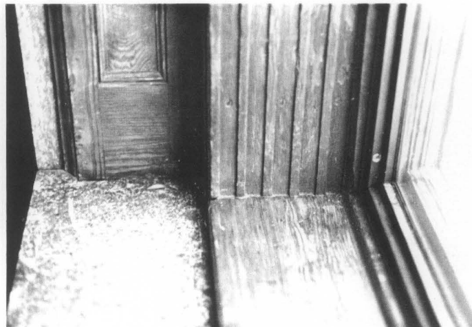
Figure 8. The decorative jamb panel on the left and the interior shutter tracks were unaffected by the installation of the interior storm window shown on the right. Photo: Charles E. Fisher
