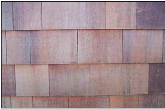
Figure 13. Shingles treated with tinted water-repellent preservative.
