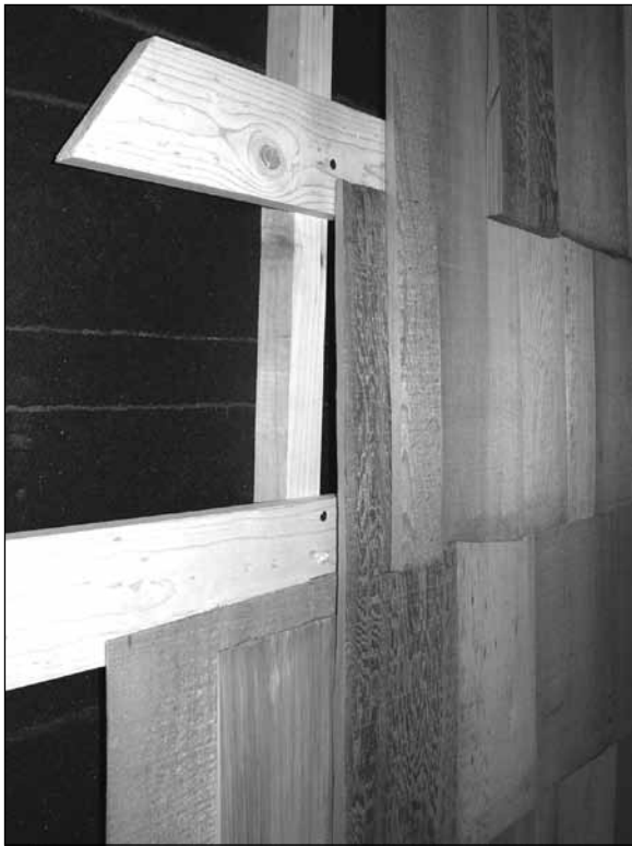
Figure 8. Rain screen technique.
