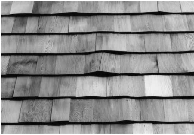
Figure 7. Buckling of shingles installed with insufficient gap.
