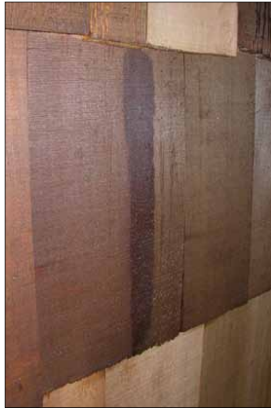
Figure 16. An example of a lap mark from improper application of a semitransparent stain.
