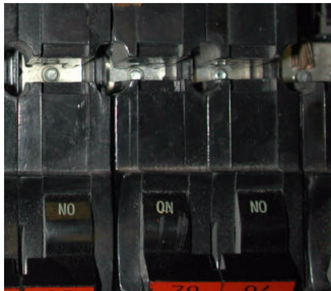
FIGURE 5 - THE ENDS OF THE SCREWS HOLDING THE STAB SOCKET PLATES ARE VISIBLE BETWEEN THE TWO ROWS OF BREAKERS. THIS IDENTIFIES IT AS A PANEL OF THE TYPE SHOWN IN FIGURE 2-C
