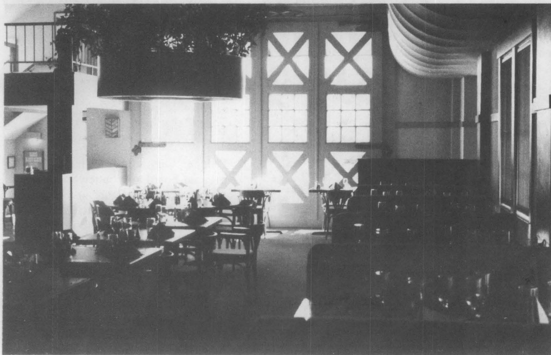
Figure 7. Replacing the tongue-and-groove boards with glass opened up the former fire truck bay while retaining the character of the doors. Photos: Chip Kaufman
