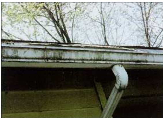
Figure 6. Sooty mold growth on house rain gutter located below a silver maple tree.
