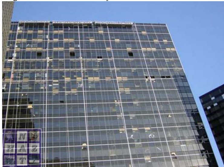
Figure 6 West face of 1250 Poydras.
