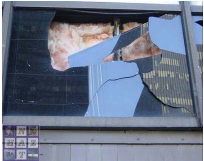
Figure 7 Broken window on north face of Hyatt Regency Hotel, likely caused by missile impact.
