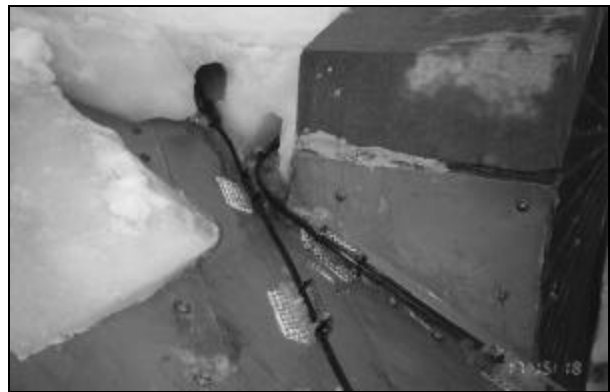
Figure 12. Electric heaters can create tunnels, which limit ponding behind ice dams on roofs.
