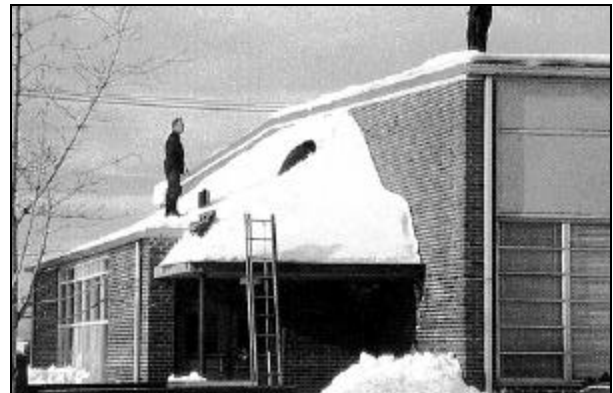
Figure 4. The peak snow load of this drift was 130 psf. The ground snow load at the time was 20 psf, and the snow load on the upper roof was 15 psf.
