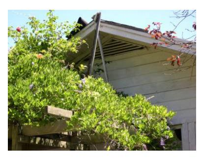
In addition to information regarding ember and flame intrusion resistance, you should also be looking at available air flow information. This is normally given in 'percent net free area' and provides information on how much area the wire (or other device(s) used in the vent design) is occupying. For comparison purposes, " mesh screen has a net free area of 81%. 1/8' and 1/16' mesh screen have net free areas of 75% and 71%, respectively. Screening with smaller openings uses smaller diameter wire.
