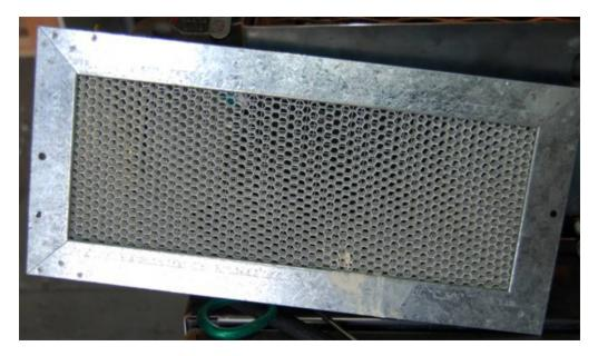
The <u>Fireguard vent</u> uses screening and a fused-link. The fused-link device is shown in the photo inset. Activation of the fused-link causes a metal door to close.
