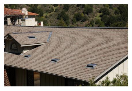
There are several kinds of vents. In crawl spaces two or more vents, to allow for cross ventilation, are used and should be located on at least two opposing walls. In attics and cathedral ceilings, air inlet and air outlet vents are used. Inlet vents are usually in the eave and soffit area. Outlet vents are placed at or near the ridge line of the roof. A ridge vent and through-roof vents can be seen on the roof of the building shown here.
